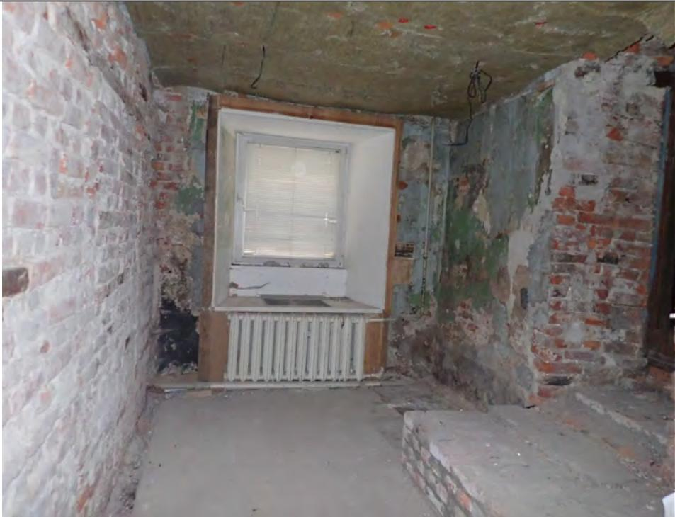
A photograph of the interior of a room. The walls are made of brick and are partially covered with peeling paint and green mold. There is a window with white blinds and a white radiator below it. The floor is concrete. |
