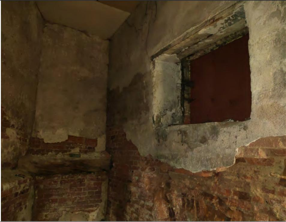
A photograph showing the interior of a room. The walls are heavily damaged, with large sections of plaster missing, revealing the underlying brickwork. A window opening is visible on the right side, with a dark interior. The floor is also damaged and uneven. |
