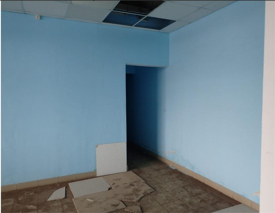
A photograph showing the interior of a room. The walls are painted a light blue color. The floor is made of dark tiles, many of which are broken and missing, revealing a concrete subfloor. A doorway is visible in the background, leading to another room. The ceiling has a grid pattern with some missing sections. |
